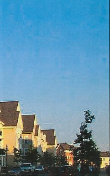
Using the IBC construction Type Vb (5b) R-2 will restrict the height to three stories and a relatively small area without a fire wall but has few difficult fire proofing requirements and fewer run-ins with approvals.
