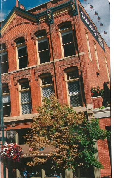
Using the IBC construction Type Va (5a) B business will raise the height to four stories (rarely seen above two) and allow enough area for a one or two office company without a fire wall.
