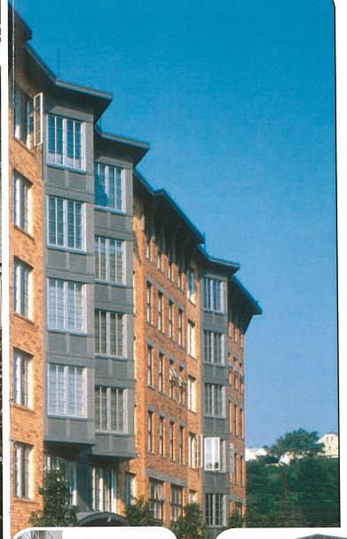
Using the IBC construction Type Ib (1b) R-2 will raise the height to eight stories and a maximum of 75' to the top landing to avoid high-rise fire safety conditions. This is however a common single use building type with time tested construction methods and traditional Euclidian zoning.
