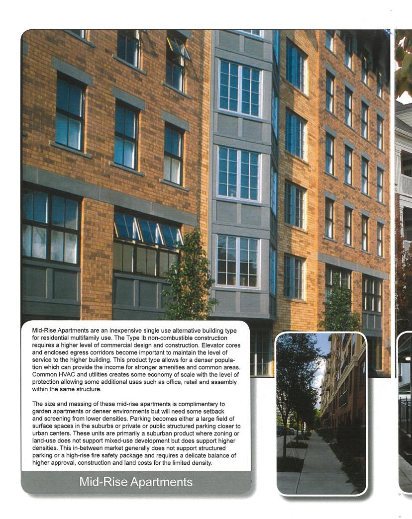
Using the IBC construction Type Va (5a) R-2 wrapped around a Type I S-2 garage will restrict the height to four stories, will restrict allowable area without a fire wall and has some difficult fireproofing conditions but is a very common separated construction type that is easily understood by jurisdictions.
